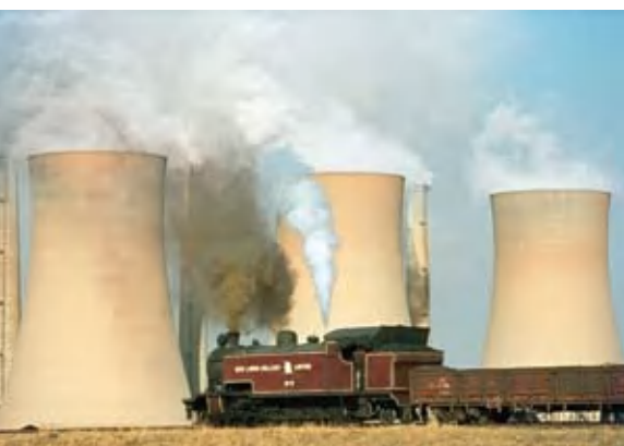
Figure 4.40 An example of a coal-fired power station
