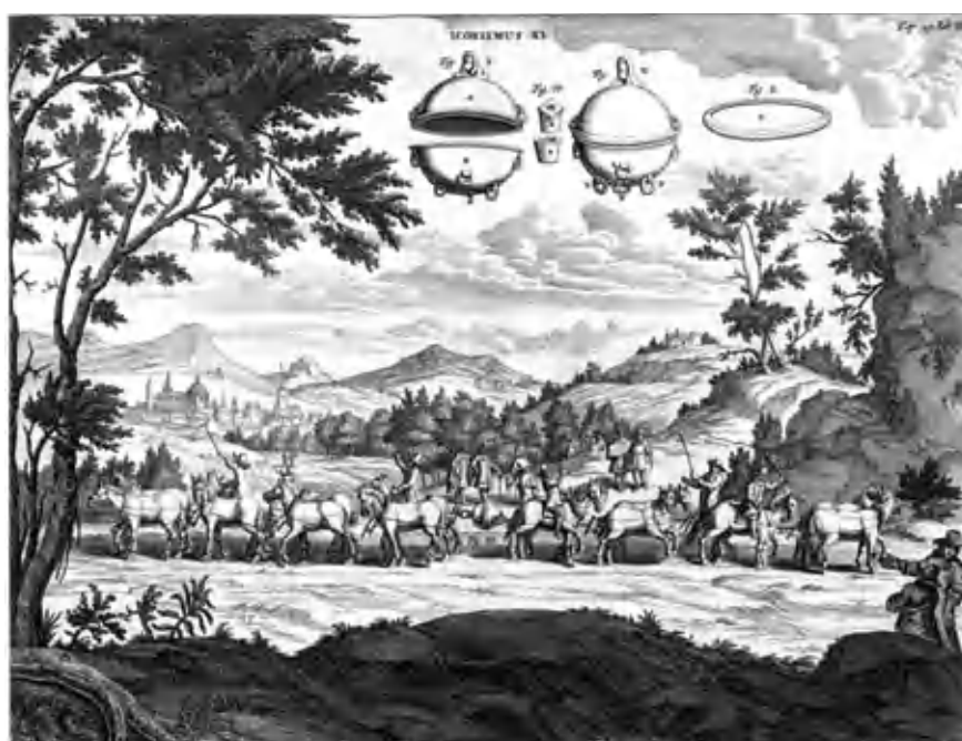
Figure 6.11 Teams of horses could not pull the hemispheres apart.
