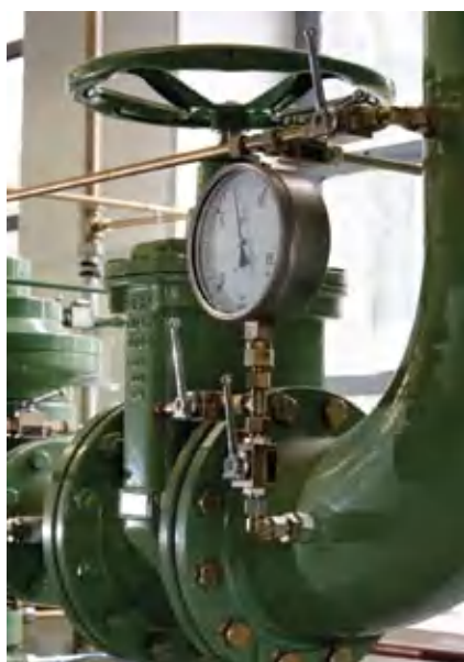
Figure 6.42 A manometer being used
