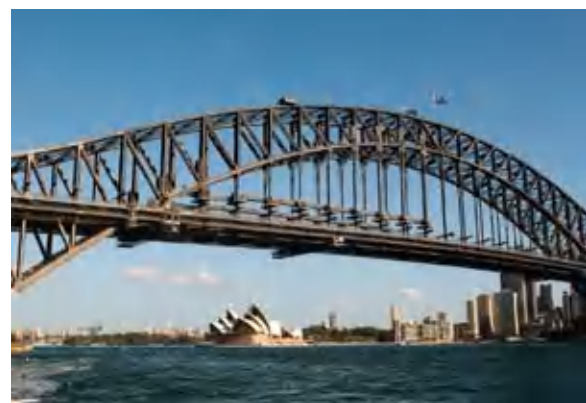
Figure 7.28 The Eiffel Tower in Paris and the Sydney Harbour Bridge were constructed using hot riveting.
